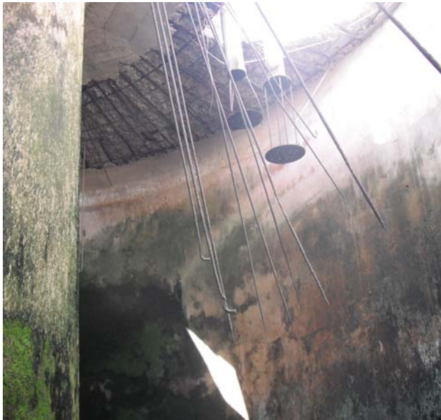
Fig.8: Broken roof slab and polluted overhead water tank.
