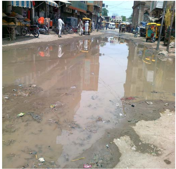
Fig.9: Storm water standing in the street.
