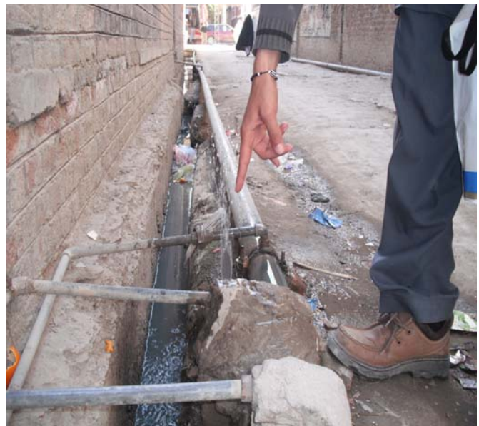
Fig. 10: : Bare leaked water supply mains lying at the banks of the sewer
